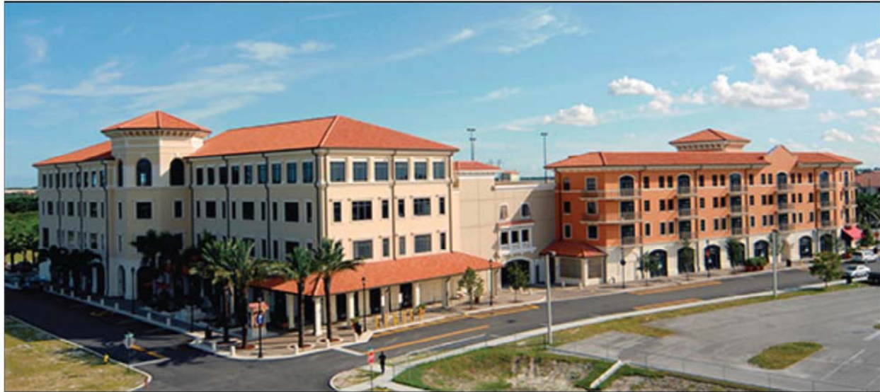
Construction is underway on Miramar Town Center, a 54-acre project with a new city hall and residential, retail and office space.
